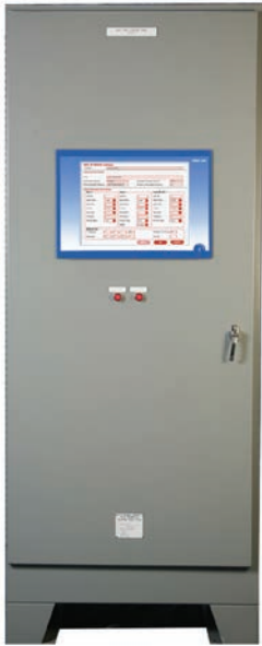
Figure 1.1 Touch 1500 mounted in the NGC-40 panel
